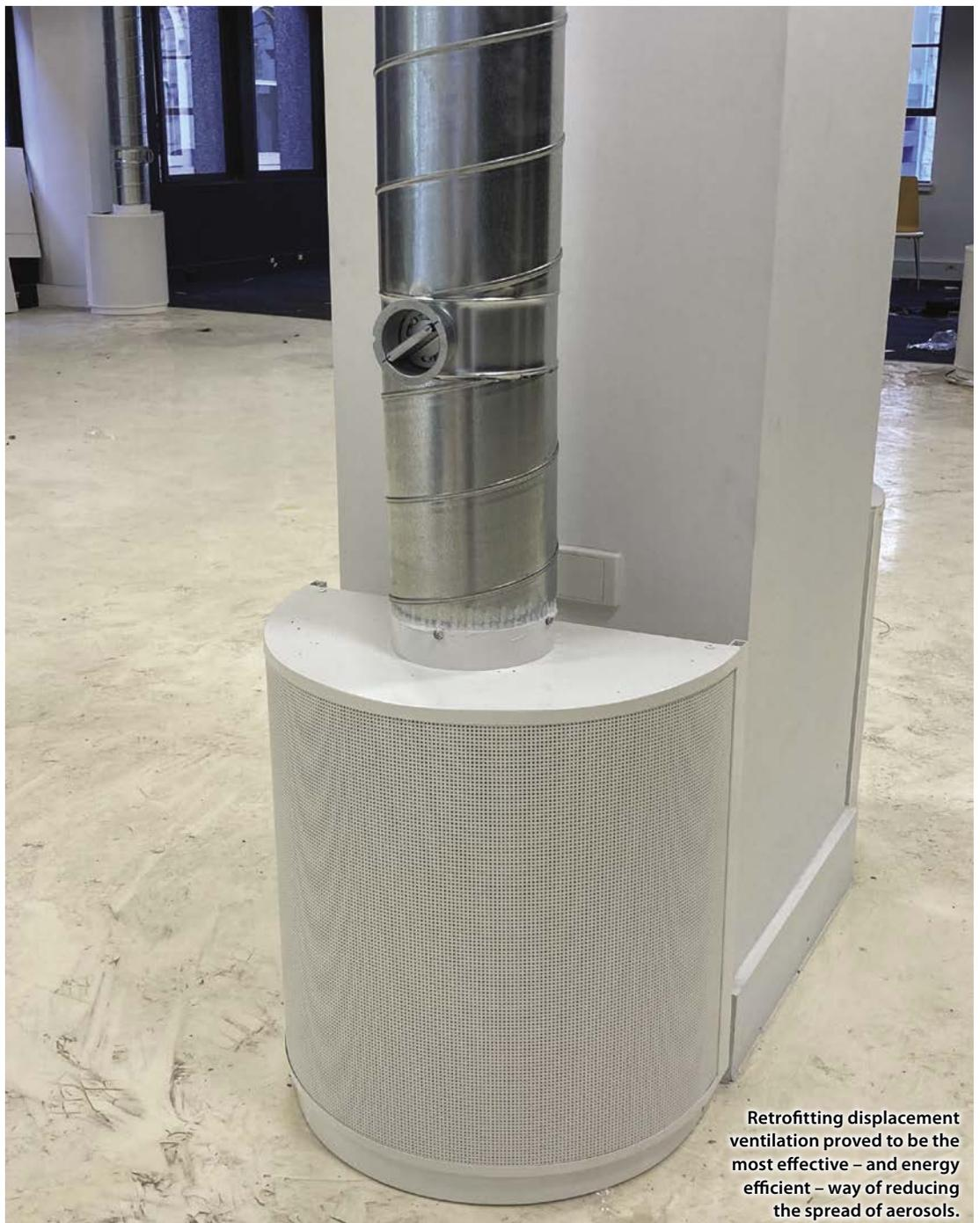
**Retrofitting displacement ventilation proved to be the most effective – and energy efficient – way of reducing the spread of aerosols.**
